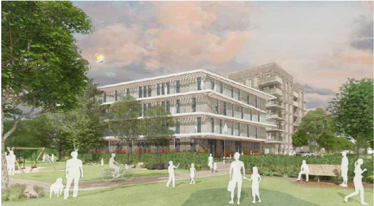
View of Building 2 from the park
